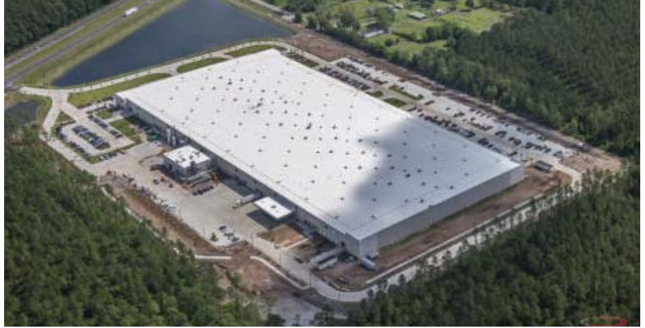
GE Oil & Gas recently decided to fully occupy this 510,443 square foot spec in Jacksonville's Cecil Commerce Center, developed by Hillwood Development, and bring about 500 high-skilled jobs to the city.
